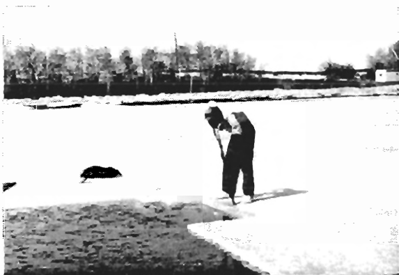
Fig. 7 Hand-sawn finishing cuts complete the beam specimen cutting procedure.
