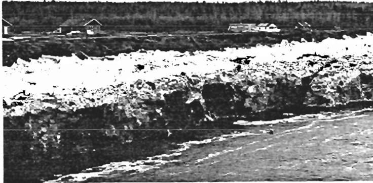
Figure 1. Shear walls remaining after ice jam release. Walls are approximately 8 m high and are a good indicator of ice jam thickness.
