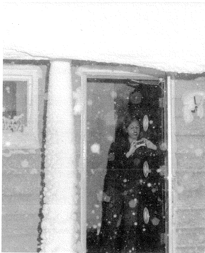
Figure 2. Evening of 30 January 1972. Snow overhangs are up to 1 m (about 3.3 ft). Snowing lightly. Vertical post is 9.6 × 9.6 cm and heavily encrusted with snow. This kind of sticking is common during windy lake-effect conditions, and is helped by supercooled water. This soon freezes.
