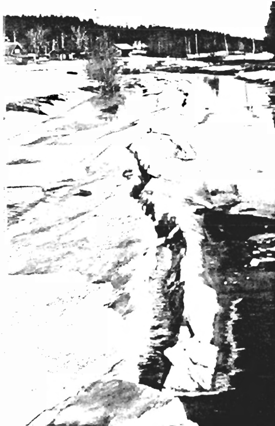
Fig. (3) Single Longitudinal Crack and Uplifted Strips Due to Rise in Water Level. Channel Width = 10 m (Courtesy of E. Kuusisto/Beltaos, 1985)
