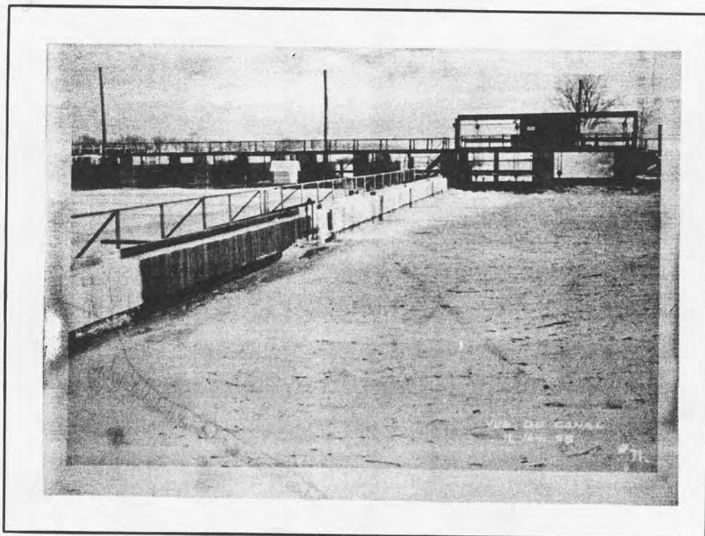
No. 4 - Downstream view of canal, showing gates, hoisting machinery and shelter for meteorological instruments.
