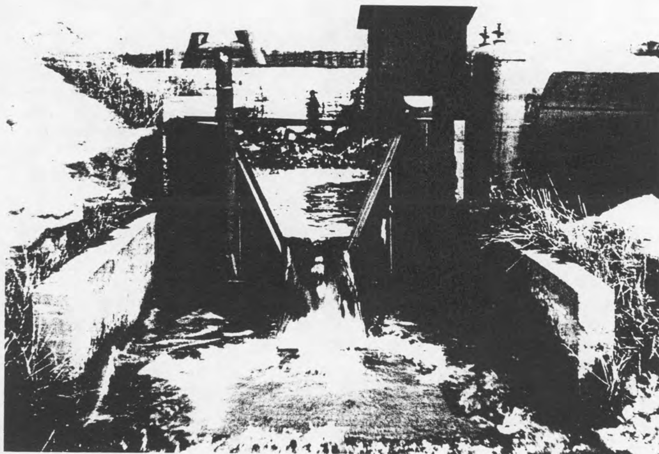
Figure 1. --Type H Rate Measuring Flume Used on Experimental Watersheds
