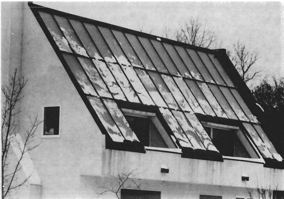
Figure 5: Snow Sliding off Steep Collectors
