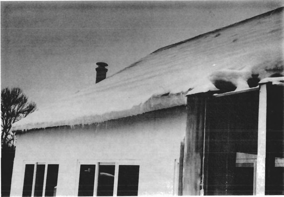
Figure 6: Snow Retention on Shallow Collectors
