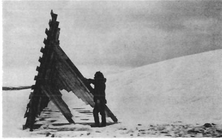
Fig. 2. Wyoming highway 3.66 m snow fence and designer Dr. Ronald Tabler. (Note significant upwind drift.)
