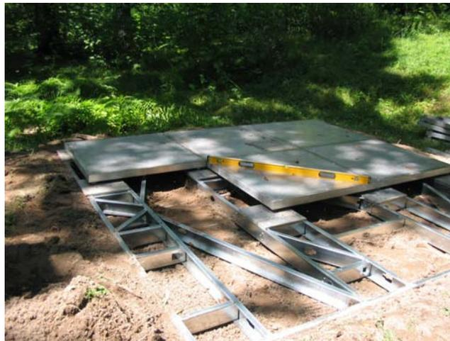
Figure 3. Installation of CRREL unit with modified sub-frame, January 2009
