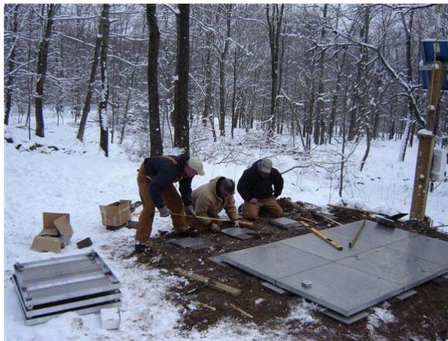
Figure 1. Installation of CRREL/NRCS Model SWE 001 Snow Water Equivalent Sensor, January 2007
